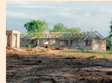
Baufortschritt in Kilifi
